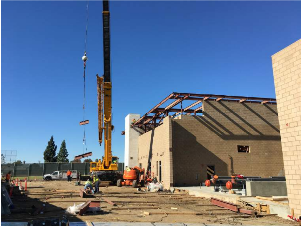
Install second floor decking and roof steel (CUP)
