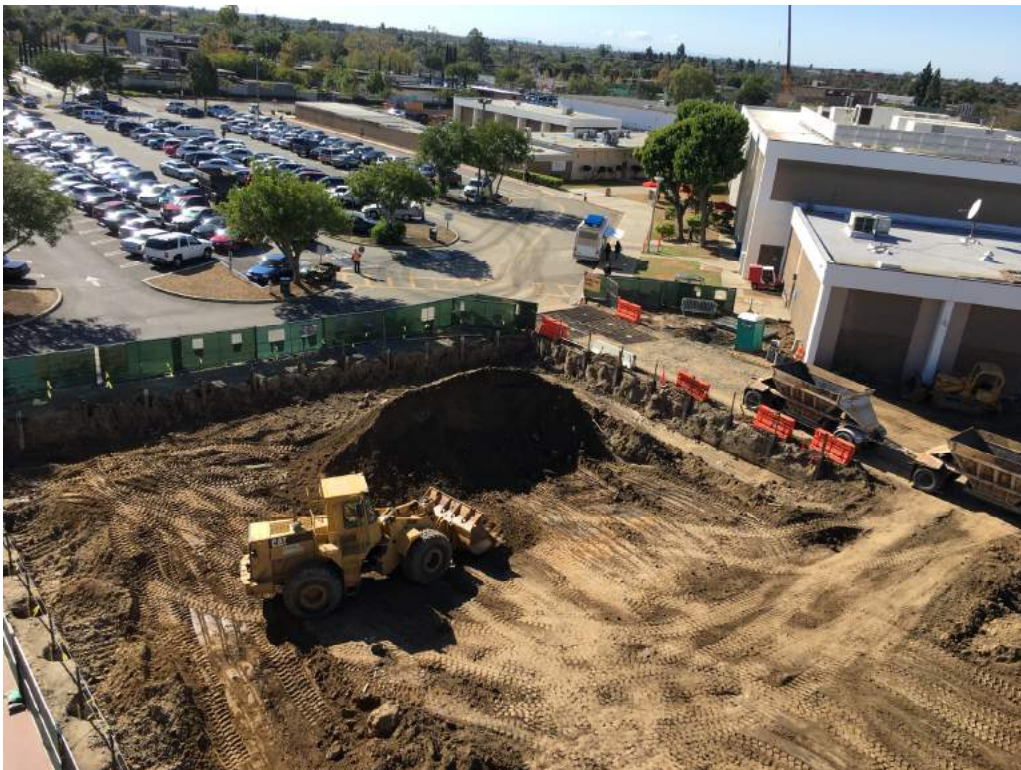
Shoring and Excavation (Amphitheater)
